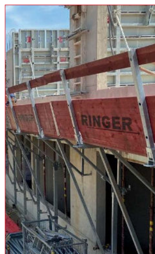
3S concreting platform
