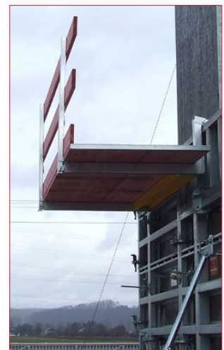
Concreting platform "L" for System 2000
